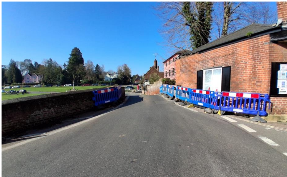
Current view of Finchingfield Bridge prior to repairs caused by vehicle damage
